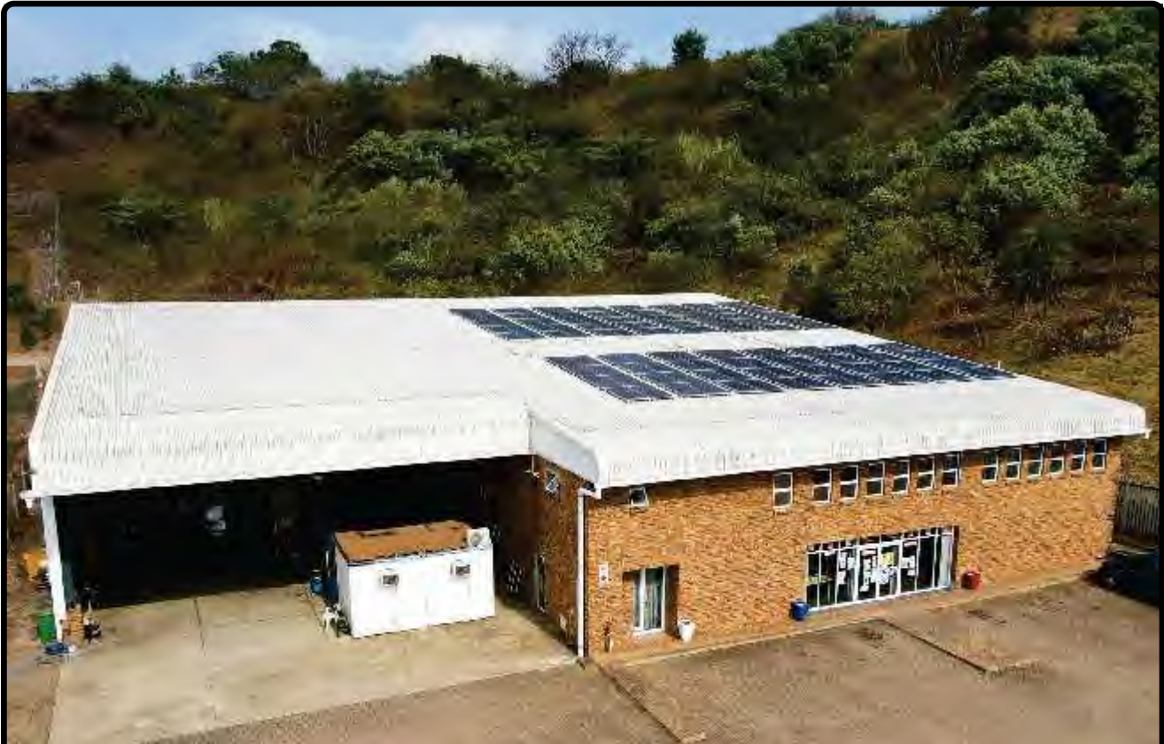
Moto-Ward Distribution Centre New Germany, KZN, South Africa
